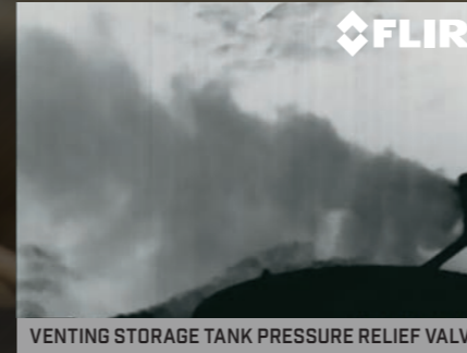
VENTING STORAGE TANK PRESSURE RELIEF VALVE
