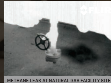
METHANE LEAK AT NATURAL GAS FACILITY SITE
