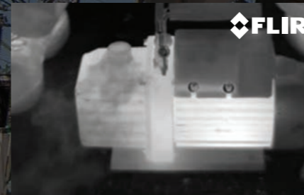
A/C COMPRESSOR - INFRARED IMAGE
