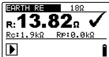
Figure 5.35: Example of earth resistance measurement result
