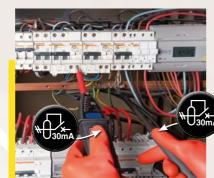
By simultaneously pressing the double command, you can cause a fault current sufficient to trip the RCD to flow through a low-impedance load.
